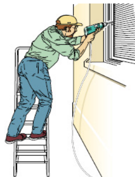
Figure 2a Incorrect - steps side-on to work activity
